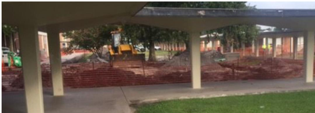
"The high groundwater table on the coast has resulted in hot soil and the piping system for the school has seen many repeated repairs for corrosion."
