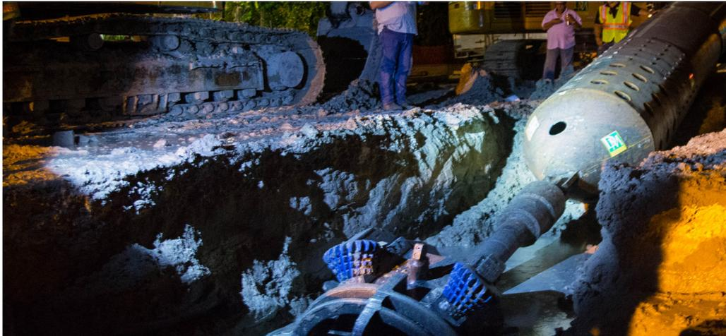
ISCO supplies HDPE for the longest 54-inch HDD pull on record.
