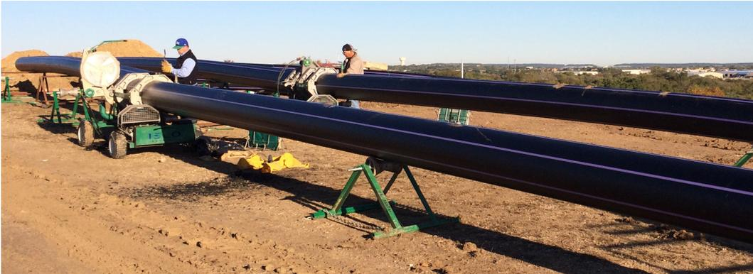
Sliplining high-density polyethylene makes an aging water line useable again.
