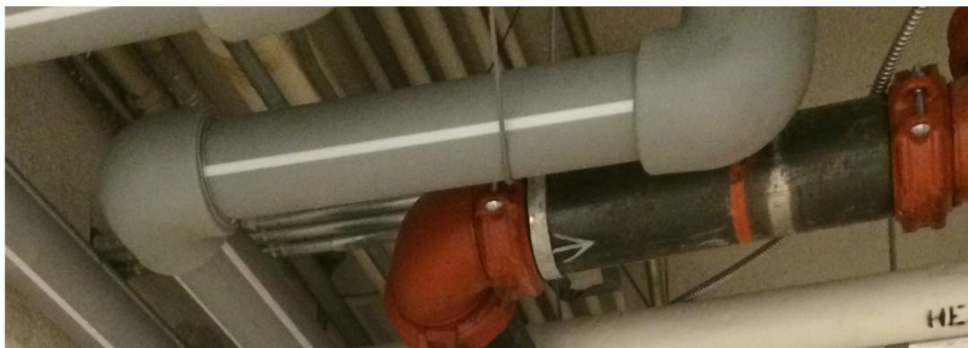
"PP-RCT is connected via heat fusion, a process of heating and joining pipe ends under pressure."
